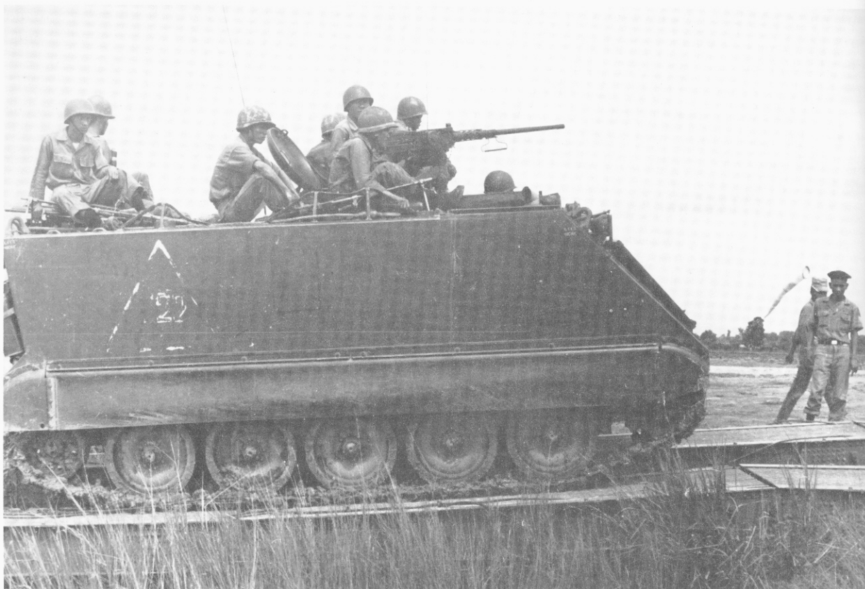
An M113 of the 7th Mech. Rifle Co. spans a watercourse by means of improvised bridging during one of the first operations in the Mekong Delta. (US Information Service)
