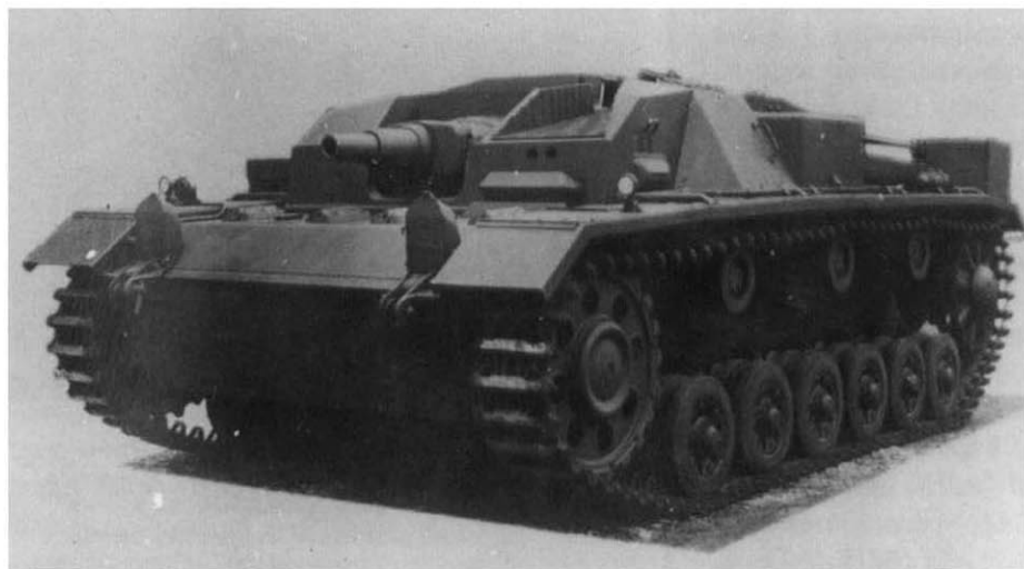
The first Sturmgeschütz Ausf.A was delivered by Daimler-Benz Werk 40 in Berlin in January 1940. This front three-quarter view clearly shows the narrow track and wheels. The entire order for 30 Ausf.A in the 1.Serie had been produced by June 1940. (National Archives)
