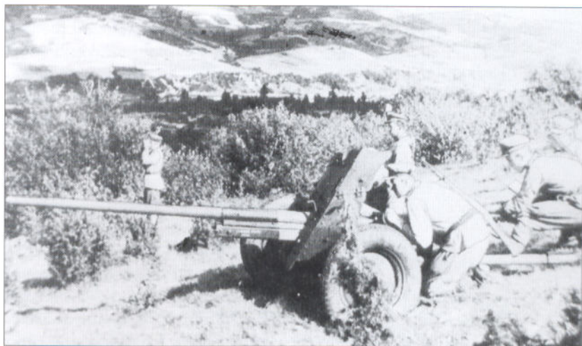
The Soviet 45mm M1942 AT gun partly replaced the 45mm M1932 as well as 37mm guns. The 45mm began to be replaced by the 57mm ZiS-2 in late 1943, but earlier models remained in use. Its long barrel coupled with a new high velocity round made the 45mm a reasonably effective weapon for its calibre. The USSR was the only country to use 45mm guns.
