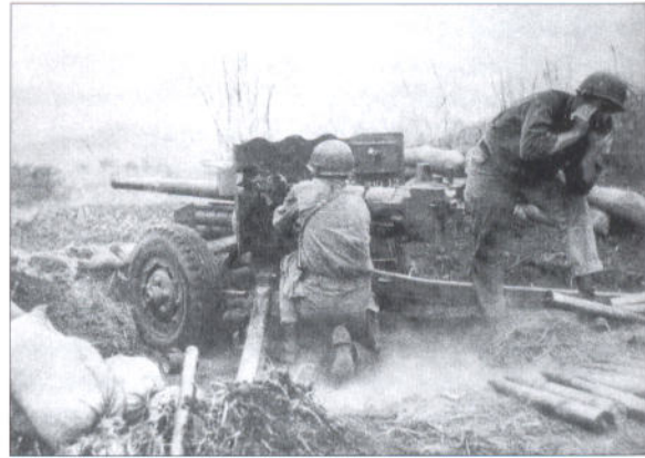
A US 57mm M1 AT gun in 'full battery'. The M1 had an artillery-type hand-cranked traverse rather than the shoulder traverse of the British 6-pdr from which it was copied. The M1A2 was provided with the shoulder traverse, however – a panel beside the breech allowed the gun to be swung freely by the gun layer's weight. The wavy shield edge, retained from the British design, helped distort the shield's appearance for concealment; and note the gun's low profile.
