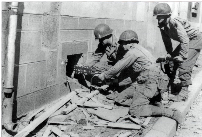
'Mouseholing': during the American operations in Brest, troops blast their way into a building through a thick exterior wall of dressed stone. In the first picture a large charge (apparently of 12x ½lb blocks) is placed carefully in a ground-level basement window – incidentally, exactly the type of position favoured for heavy weapons during the defence of city blocks. The team must have stood well back under cover during the explosion of 6lb of TNT; in the second photo a GI crawls inside the building through the hole torn by the blast. (IWM HU 94979 & 94980)
