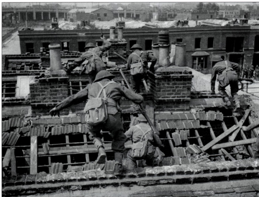
Not an exercise for troops suffering from vertigo: London Home Guards demonstrate roof-crossing at the double in a bombed-out area of terraced housing. Successfully executed, such a manoeuvre allowed an advance without using exposed streets, and allowed houses to be cleared from the attics downwards. (Imperial War Museum H 20884)
