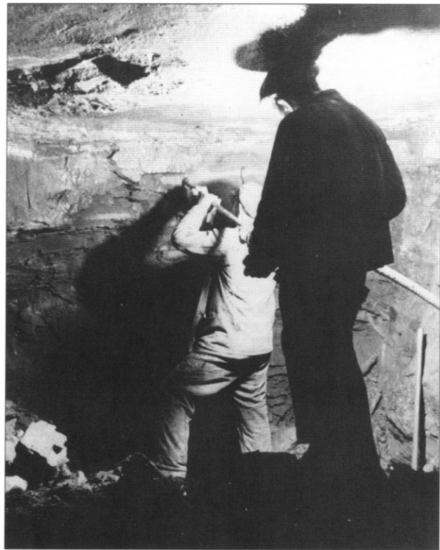
Some of the defences of the West Wall – for example the tunnel systems – were bored into solid rock. This was dirty and dangerous work and those who undertook it were given special pay and allowances. (Bundesarchiv)
