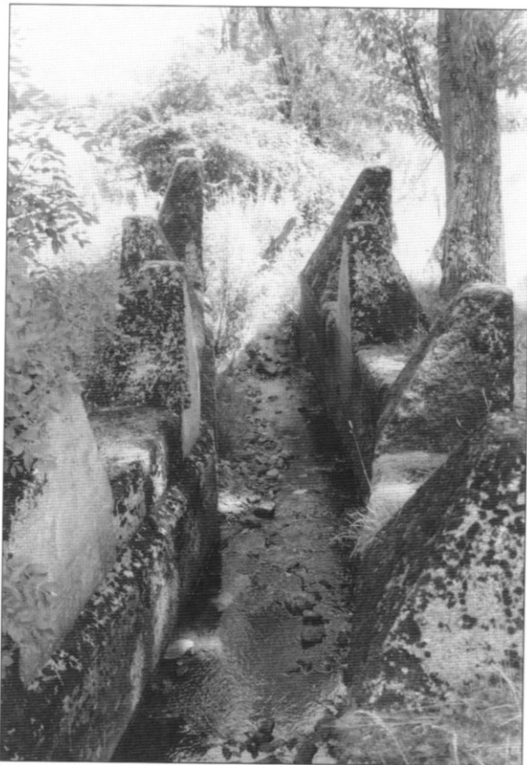
Where no natural obstacle barred the passage of tanks, engineers constructed rows of concrete anti-tank obstacles, or dragon's teeth. Inevitably, it was necessary to include breaks for roads, tracks and in this case a small stream. This obstacle is still visible and is located near the village of Lammersdorf. (Author's collection)
