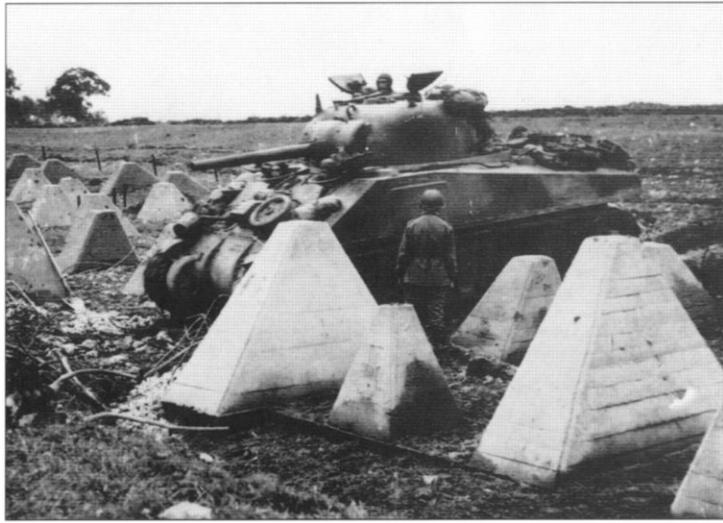
An American Sherman tank follows the path blasted by US Army Engineers during the fighting around Aachen in September 1944. The Americans tended to attack road blocks rather than sections of dragon's teeth because destroying the teeth was dangerous and time consuming. (Imperial War Museum)
