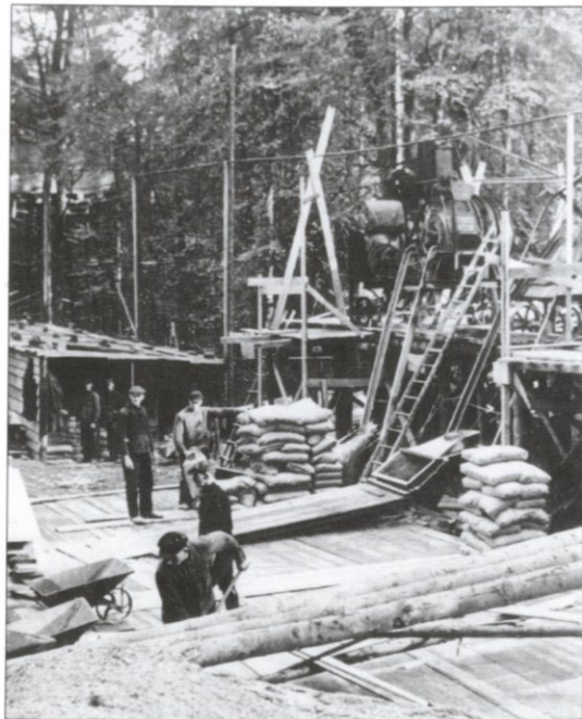
The construction of the West Wall employed the majority of the country's concrete mixers. Cement, sand and gravel were loaded into hoppers at the bottom and lifted up to the mixers which could then pour the mixture in the desired place. October 1938. (Bundesarchiv)
