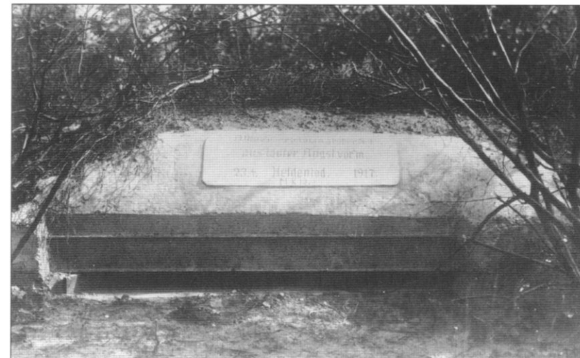
Some of the defences of the Hindenburg Line were very substantial and not that far removed from some of the more basic structures of the West Wall. This concrete and steel pillbox was built at Le Pave. The inscription reads, 'In greatest need was this built here, for a hero's death I greatly fear, 23.4.17 M.K.19'. (Imperial War Museum)
