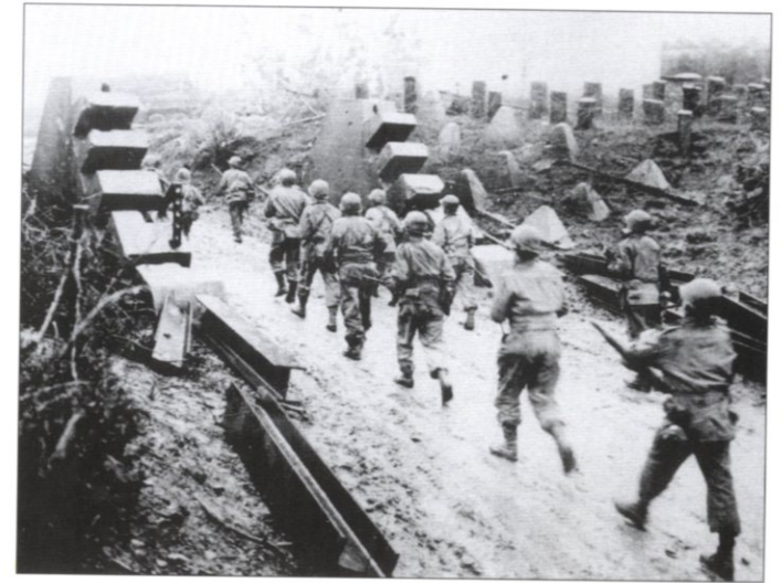
Men of the 39th Infantry Regiment (9th Infantry Division) pass through the Siegfried Line near Roetgen. In the immediate foreground are iron girders that were placed in the recesses of the trägersperre to block the road. To the sides are dragon's teeth and improvised anti-tank obstacles which are simply wooden posts rammed into the ground. (US National Archives)
