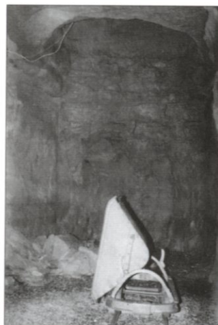
The tunnel system of the Gerstfeldhöhe was designed to have two levels – an upper or fighting level and lower or storage/sleeping level. To link the two a 68 metre high lift shaft was to be constructed. The lift was bored, but the lift was never completed. (Author's collection)
