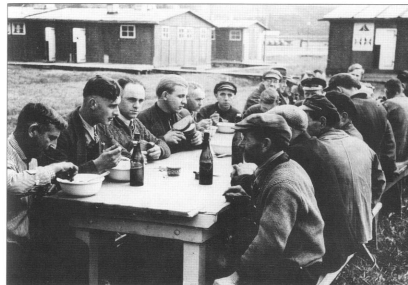
Workers on the West Wall enjoy their meal, washed down with beer, 'al fresco'. The barracks to the rear would have served as their sleeping quarters. Despite the propaganda images living conditions were difficult especially in the winter. (Bundesarchiv)
