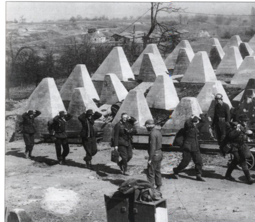
American military policeman process German POWs as they pass through a section of dragon's teeth. The pristine looking teeth appear to be of the larger type 1939 pattern which were built to counter the development of bigger more powerful tanks. The teeth to the right appear to be originals painted green to merge in with the landscape. (Imperial War Museum)
