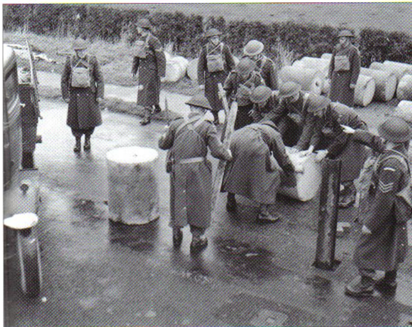
A none-too-young group of Home Guardsmen practice erecting an AT barrier during a Northern Command exercise in November 1941. At least one rail has been placed into a socket (note the socket covers) whilst heavy concrete cylinders are being positioned in threes in front of the rail. The cylinders were designed to impede the movement of a tank attempting to smash through the rails. Rubble would have been scattered about to prevent overturned cylinders being used by a tank as rollers. (IWM H 15192)
