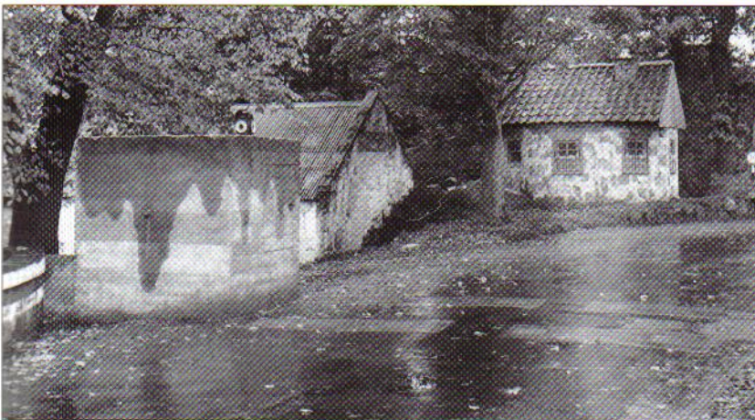
Another ingeniously camouflaged pillbox: it is a pity that the large concrete block, restricting the road width, gives the game away! To its right, sockets for steel AT rails have been fitted. This photograph was taken in October 1940. (IWM H 4774)
