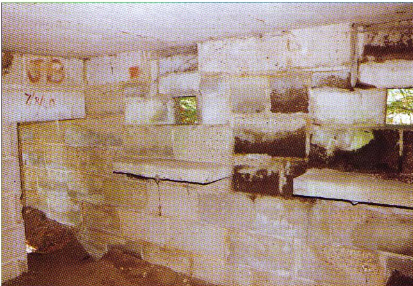
TOP One of the pillboxes built by the BEF in 1939–40 at Cysoing in their sector of northern France. This particular design was grouped in fours to cover a French AT ditch. (MO)
