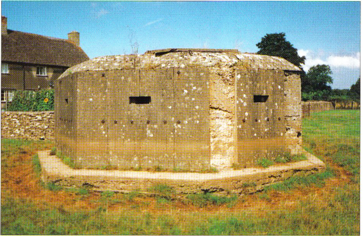
A surviving 'shell-proof' pillbox of the Bristol defences at Avening, Gloucestershire, which would have faced an AT ditch. This pillbox uses concrete panels as permanent shuttering and is based on the War Office Fortifications and Works design FW3/24 of 1940.
