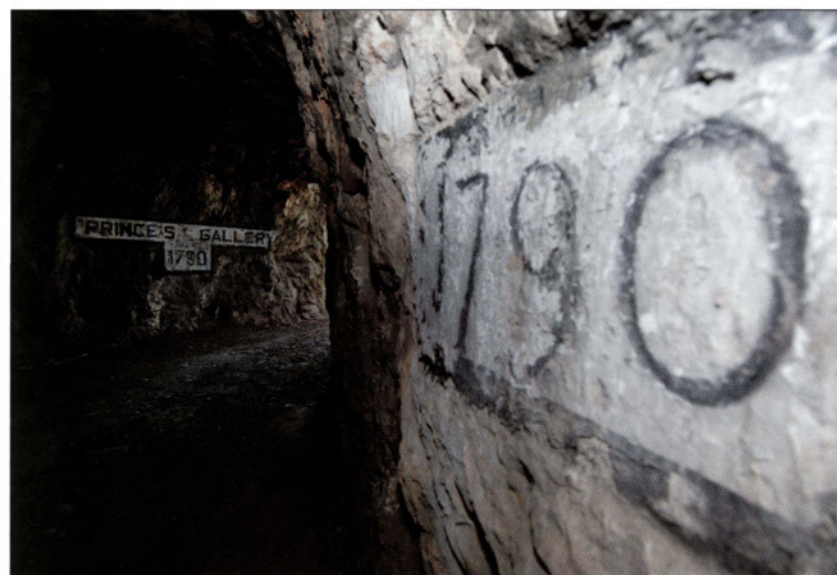
Prince's Gallery forms part of the Lines of the same name, leading to Hanover Gallery to the west. The Prince's Lines are part of the Northern Defences and run above King's and Queen's Lines, all of which flanked the landward approaches to the city. (Authors' photograph)
