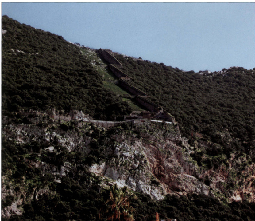
The upper section of Charles V Wall showing its 'stepped' ( en cremaillère ) disposition, which allowed each face to receive flanking fire. Note also the steep cliffs at its base, making access to the upper Rock difficult. In Bravo's time it was called the Muralla de San Benito. (Authors' photograph)
