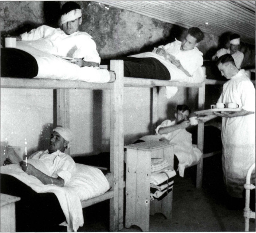
'Minor sick and wounded' were accommodated in two-tier bunks. More serious cases had hospital beds. Note the stone wall alongside the bunks. A suspended ceiling of corrugated iron sheeting protected the men from water drips and small stones that could fall from the tunnel roof. (Courtesy of the Imperial War Museum)
