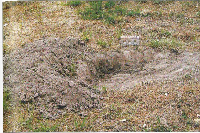
The author dug this rifleman's hasty firing position with an entrenching tool in 10 minutes to the dimensions prescribed in the Soviet manual. The thickness of the loose earth parapet would be ineffective against rifle fire. For scale, the brick measures 9 x 19cm. (Author's collection)
