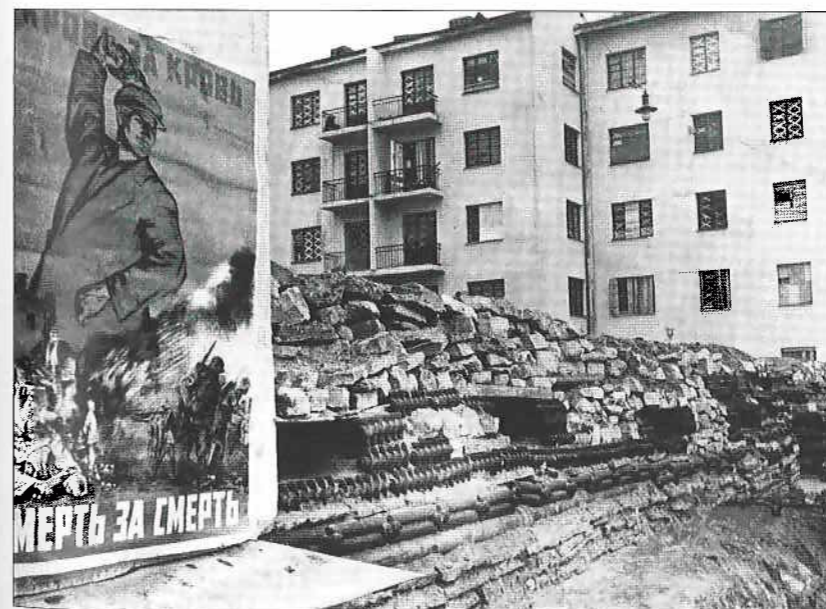
This street barricade with firing embrasures was built between two apartment blocks. Tank tracks have been incorporated into the rock and sod barricade. A shallow anti-tank ditch fronts the barricade, from which the building materials were excavated. Besides a firing position, it presents a formidable anti-tank barrier. Note that some apartment windows have been barricaded with concrete blocks, and possessed embrasures. (RGAKFD)
