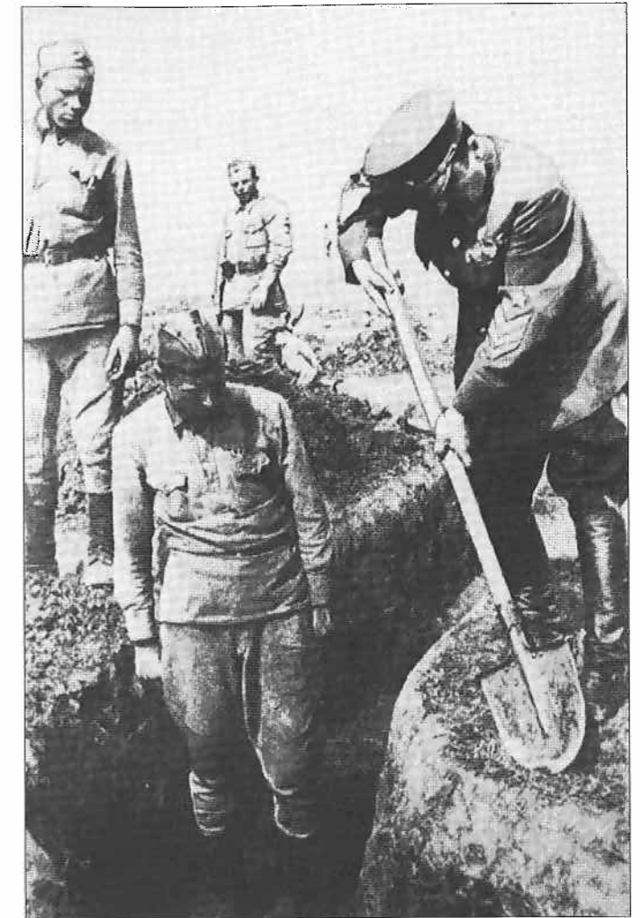
A posed photograph, no doubt, of a general assisting with the tidying up of a crawl trench. Both square- and round-nose, long-handle shovels were issued. An elbow rest lip was provided behind the parapet for rifle firing. (Author's collection)
