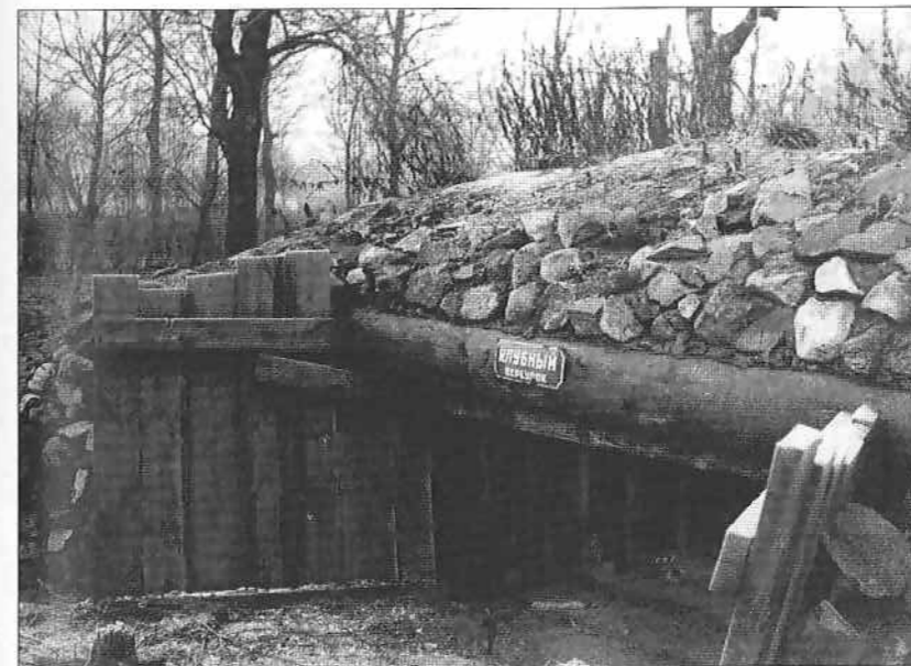
This heavily constructed machine-gun bunker is built of logs, covered with earth, and topped with a layer of rocks. The exposed rock covering and large-plank embrasure make it conspicuous. (RGAKFD)
