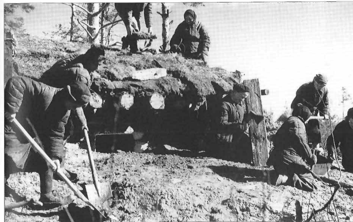
Impressed civilians complete a heavy machine-gun bunker. Camouflaging sod is being laid on the bunker's roof. While the bunker is large, note the small size of the rock-faced embrasure. Civilians were directed by engineer officers. (RGAKFD)
