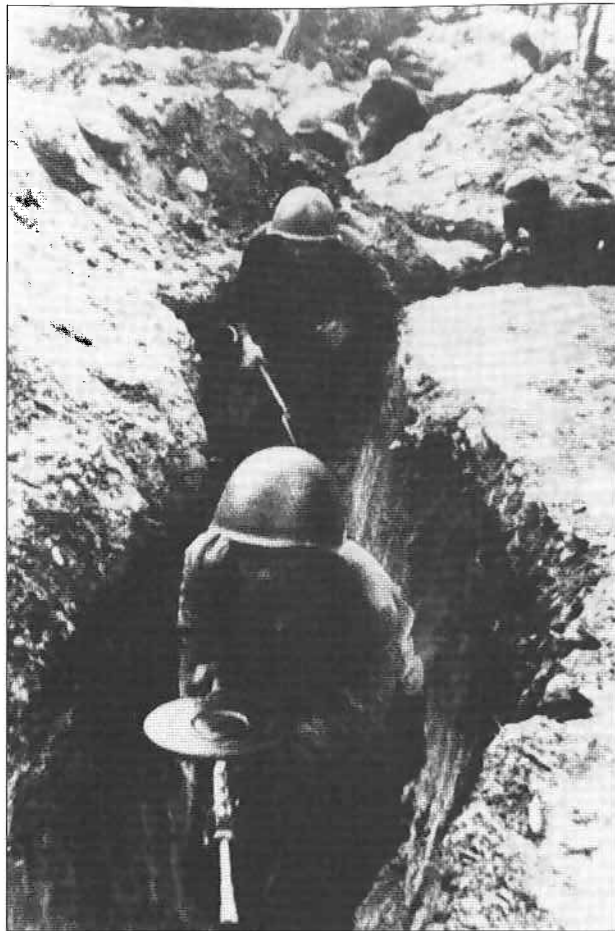
A crouching-type communications trench outside Leningrad. Note that in this instance the spoil has been thrown to the enemy side along at least part of the trench to provide a higher parapet. A 7.62mm DP-armed machine gunner is in the foreground. (Author's collection)
