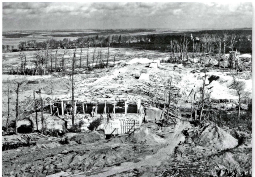
The Wasserwerk St. Pol at Siracourt was the most heavily attacked of the heavy sites. Although the concrete work was largely complete, as is evident from this Allied intelligence photo from the summer of 1944, the excavation of the interior earth core had not progressed very far before the bombing halted final construction. (NARA)
