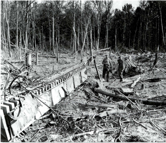
A thoroughly smashed V-1 launch site, presumably after an air attack. The Walter catapult has been broken into several pieces and is being examined by an Allied technical intelligence team. (NARA)
