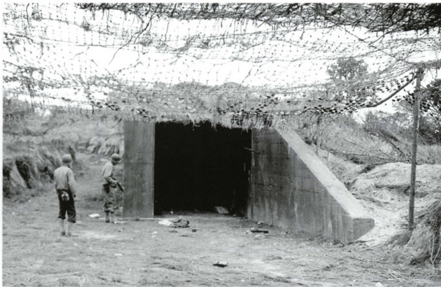
The threat of air attack led FR 155(W) to make extensive use of camouflage nets around the launch sites. This is a "ski" stowage building at one of the Abteilung IV sites near Cherbourg. (NARA)
