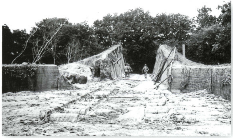
The Bois-Carré sites protected the Walther catapult with reinforced walls on either side. This is a typical example near the Chateau de Sorrelerie in the Cherbourg area, one of the batteries of Abteilung IV. (NARA)
