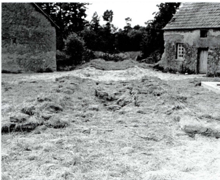
The new sites were almost invisible from the air until the Walther catapult was erected. This shows one of the launch sites of Abteilung IV on the Cotentin Peninsula abandoned after D-Day. The concrete launch pad and rails are camouflaged with hay. (NARA)
