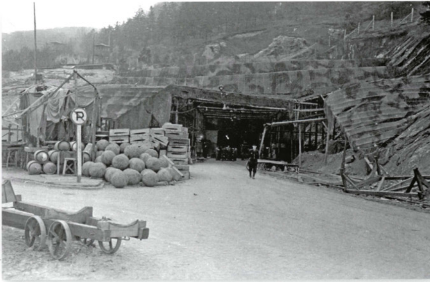
The Mittelwerke complex was so well hidden that the Allies did not bomb it. This shows one of the camouflaged entrances after its capture by the US Army in April 1945. (NARA)
