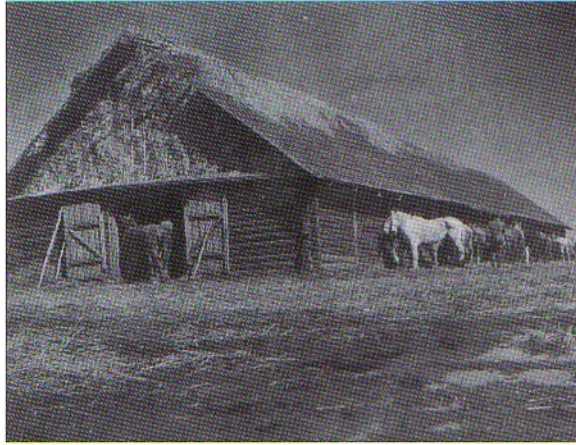
A field stable, probably in Russia. The log construction gave good protection against the cold and rain, but the risk of fire was high – note the thatch on the front gable. (Paul L. Johnson Collection)
