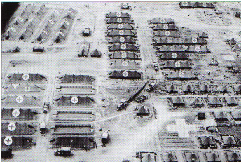
The evacuation hospital on the Anzio beachhead was hit by enemy artillery and bombs on a number of occasions. Protection was afforded to the flimsy tents by digging shallow ditches round them and using the soil to build low splinterproof walls - see the bottom left corner of the picture.
