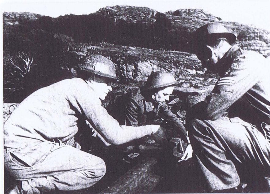
Film still showing Harry Ree (left) and Jacqueline Nearne (centre) being instructed in rail sabotage. Nearne is taping plastic explosive (PE) under the rail while Ree places a fog signal detonator on top. Several lengths of track were set up for SOE to destroy as part of the Group A paramilitary school. (IWM MH24449)
