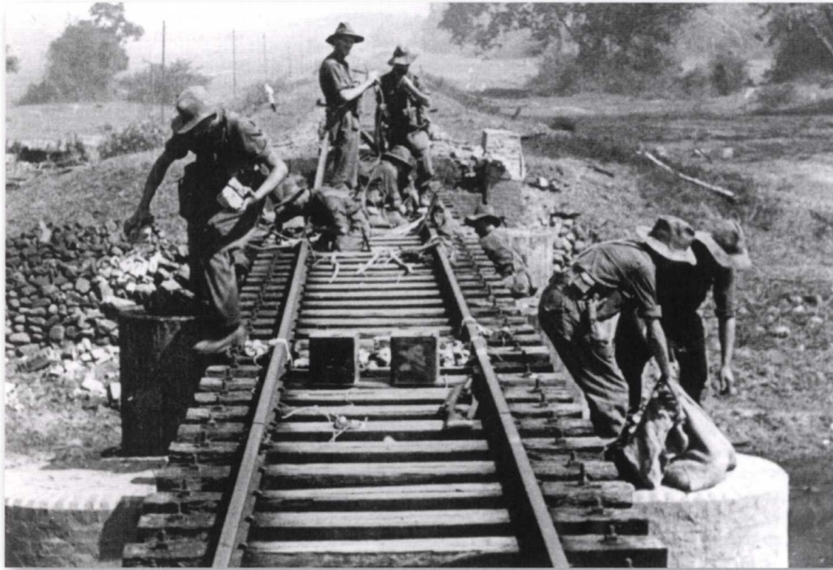
A group of Chindits on Operation Longcloth prepare a railway bridge for demolition. (SE 7921)
