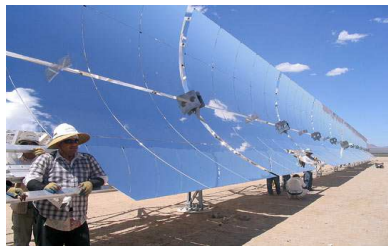
Fig. 3 Solar Power Plant
