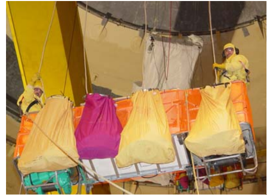
Workers positioned to paint the containment dome
