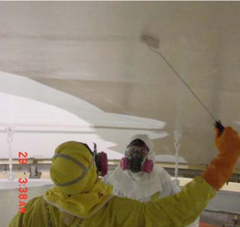
Cannon-Sline workers, applying paint to the dome of the Containment Building.
