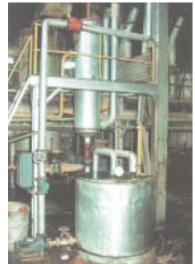
Direct Contact Heat Exchanger (DCHE) tampak luar
